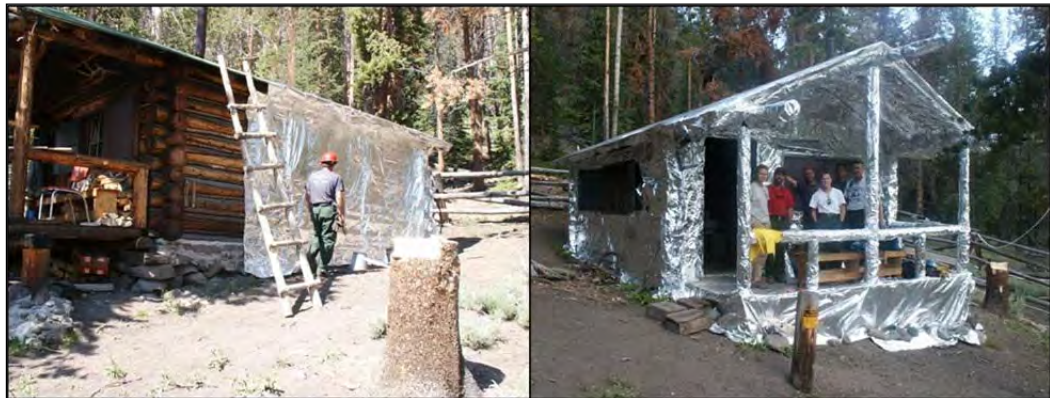
Figure 1.5. Example of one of the management strategies. The crew seen above is protecting the Venus Cabin from the LVF. This building survived. This image was adopted from the 2006 Case Review, Little Venus Fire Shoshone National Forest WY-SHF-09.
