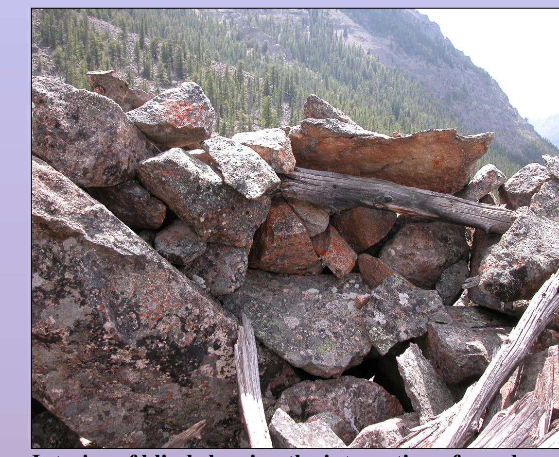
Interior of blind showing the integration of wood elements as transverse cross-beams.
